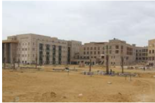
AUC New Cairo campus garden under construction, 2008
